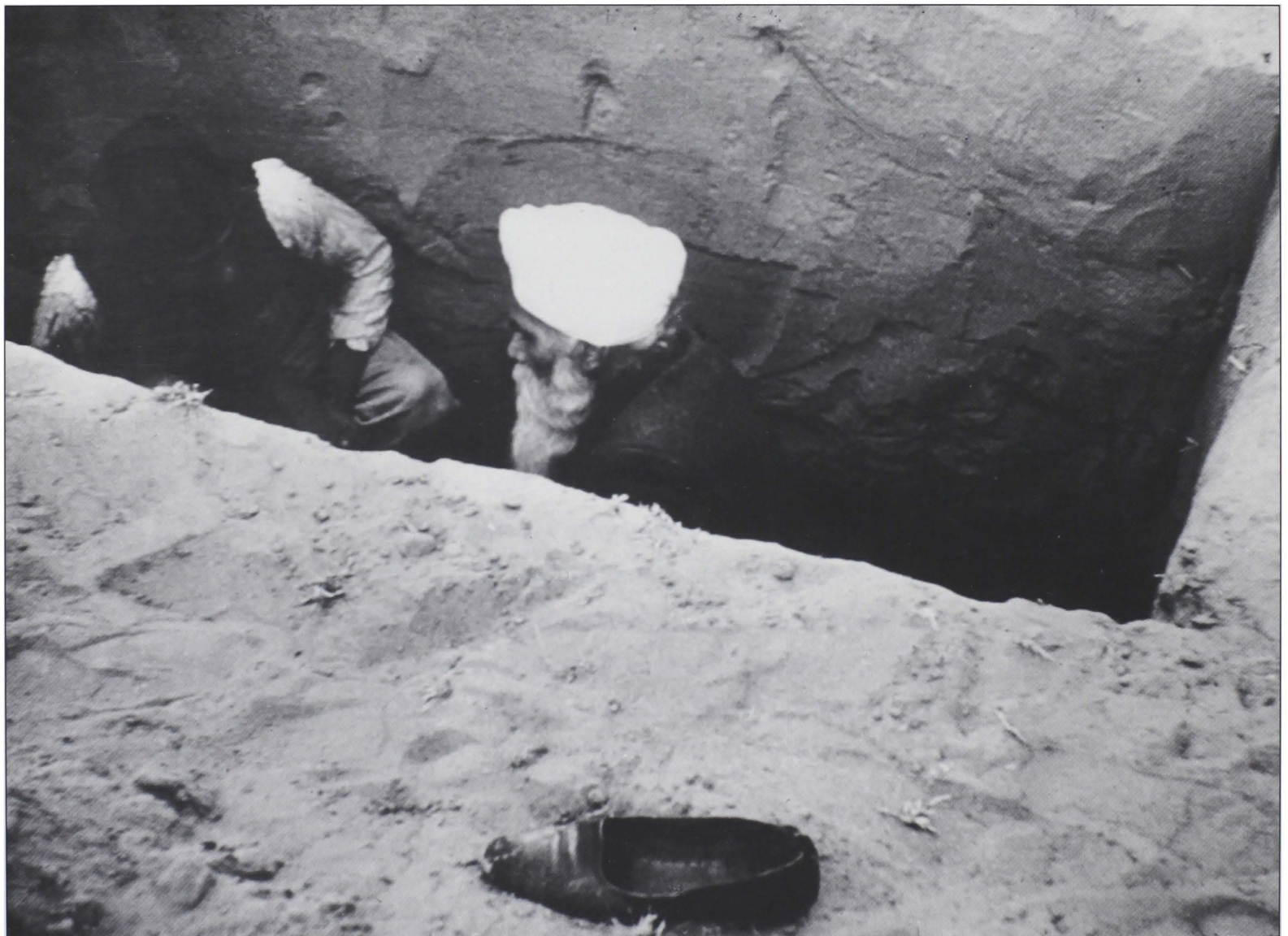
Winter 1949: Sardar Bahadur Maharaj Ji laying the foundation stone of the Satsang Ghar at Jullundur.
